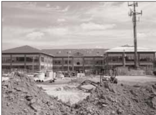
Photo of new dorms under construction
