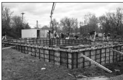
Photo: carpentry students poured the foundations and walls at homes being build on Evans Avenue.
